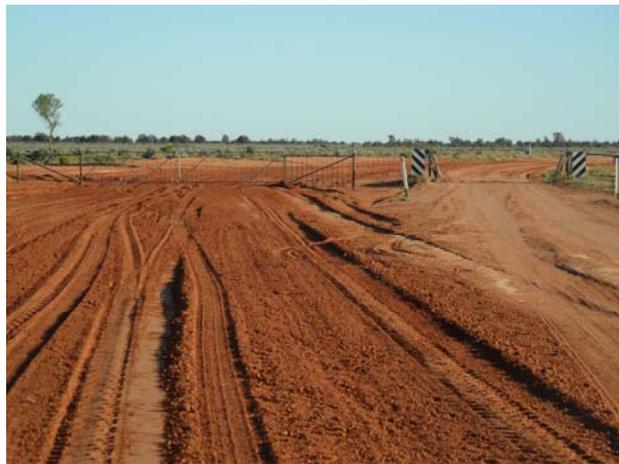
*Views of the access road upgrading work being carried out by CMC, including construction of detours for wide heavy equipment around the numerous narrow grids and gates.*
