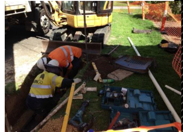
Trench cutting prior to laying new conduit
