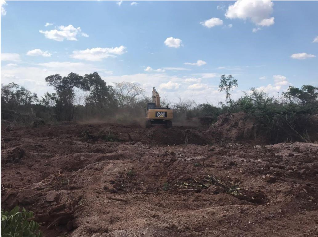
**Figure 4 - Land clearing for village construction site**
