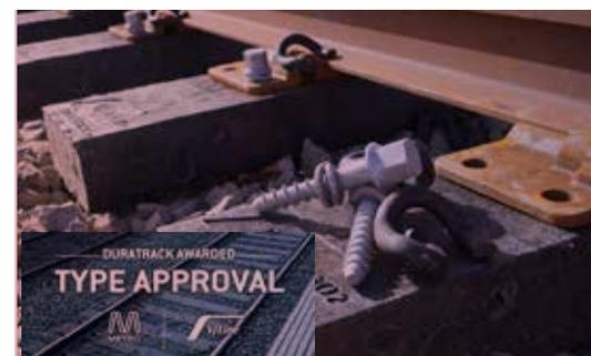
Duratrack is a sustainable railway sleeper with a 50-year life. Then, at the end of its life, it can be recycled back into another sleeper. In an Australian first, the Duratrack railway sleeper has been granted type approval for mainline use.
