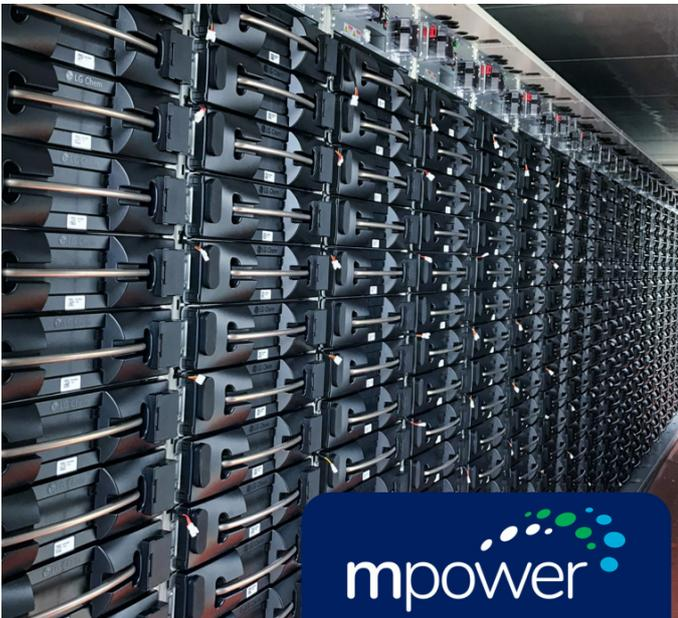
Image: A lithium-ion battery energy storage system designed and delivered by MPower
