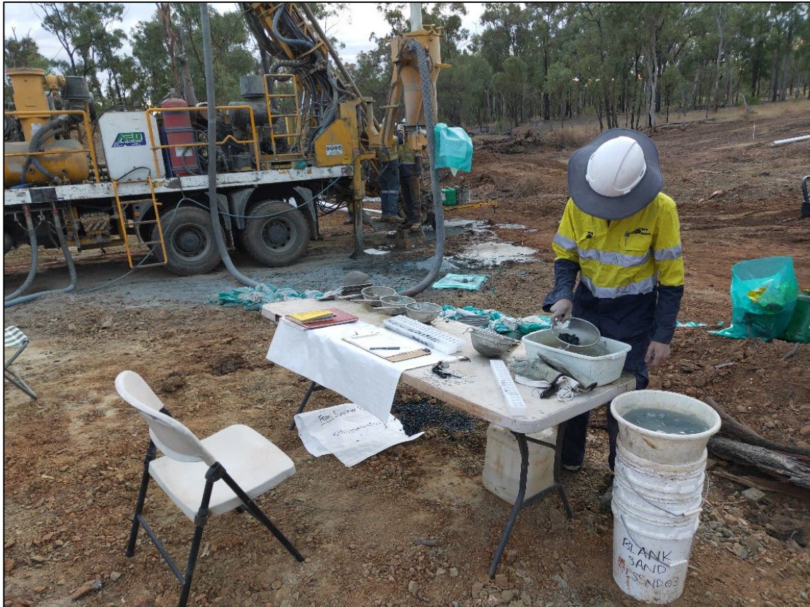
Figure 12. RC drill chips being washed in preparation for logging and chip tray storage.
