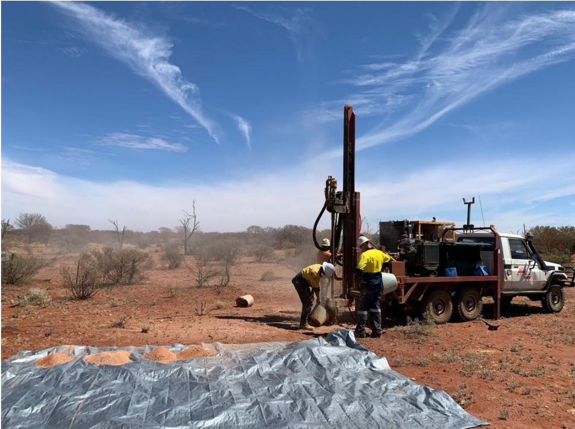
***Photo RAB Drilling Operations at Comet***
