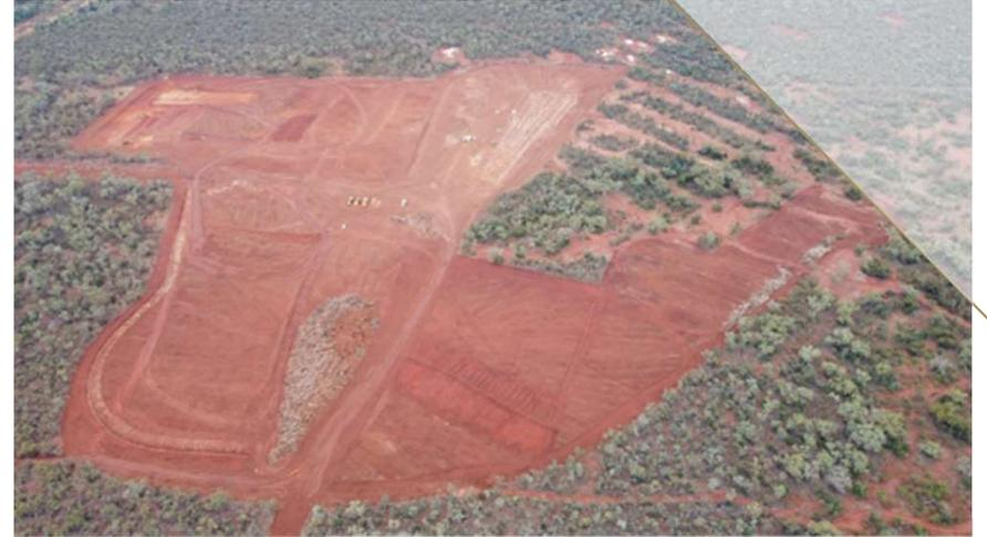
Neill Earthmoving cleared and grubbed 32 hectares of land, established access roads, and commenced excavation for the box cut.
