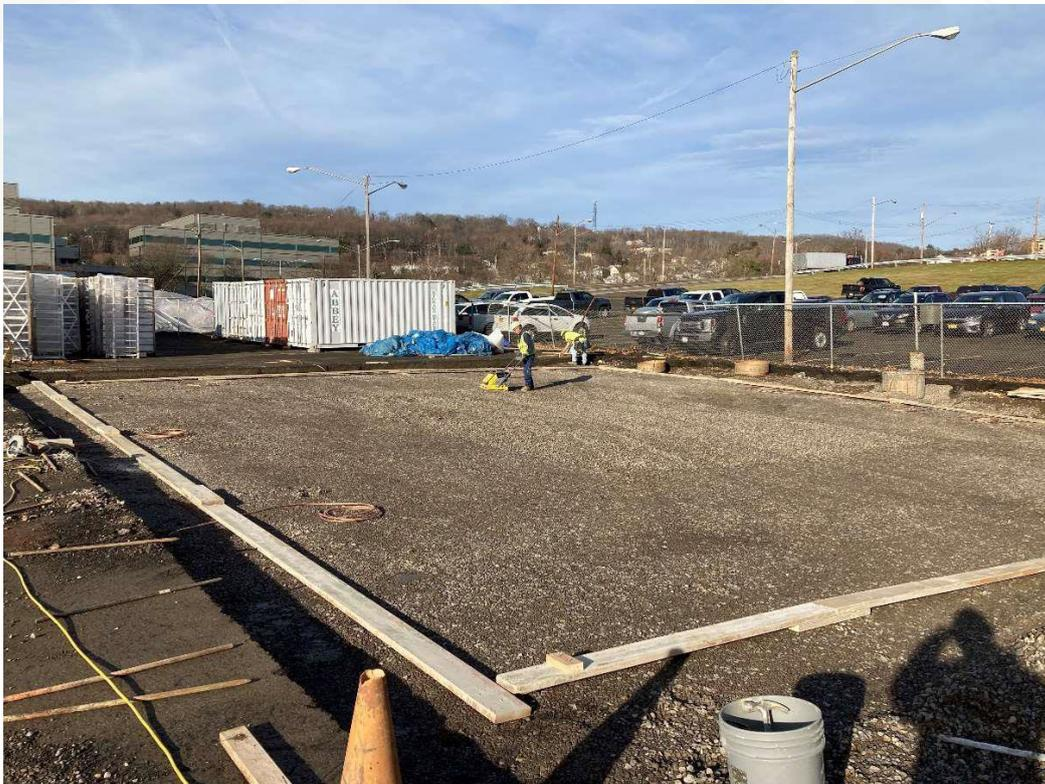
Figure 4: Exterior foundation pad preparation for Solvent Recovery System
