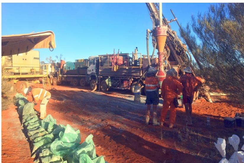
Figure 1. Bullion Drilling Company reverse circulation drill rig onsite for drilling at Soyuz
