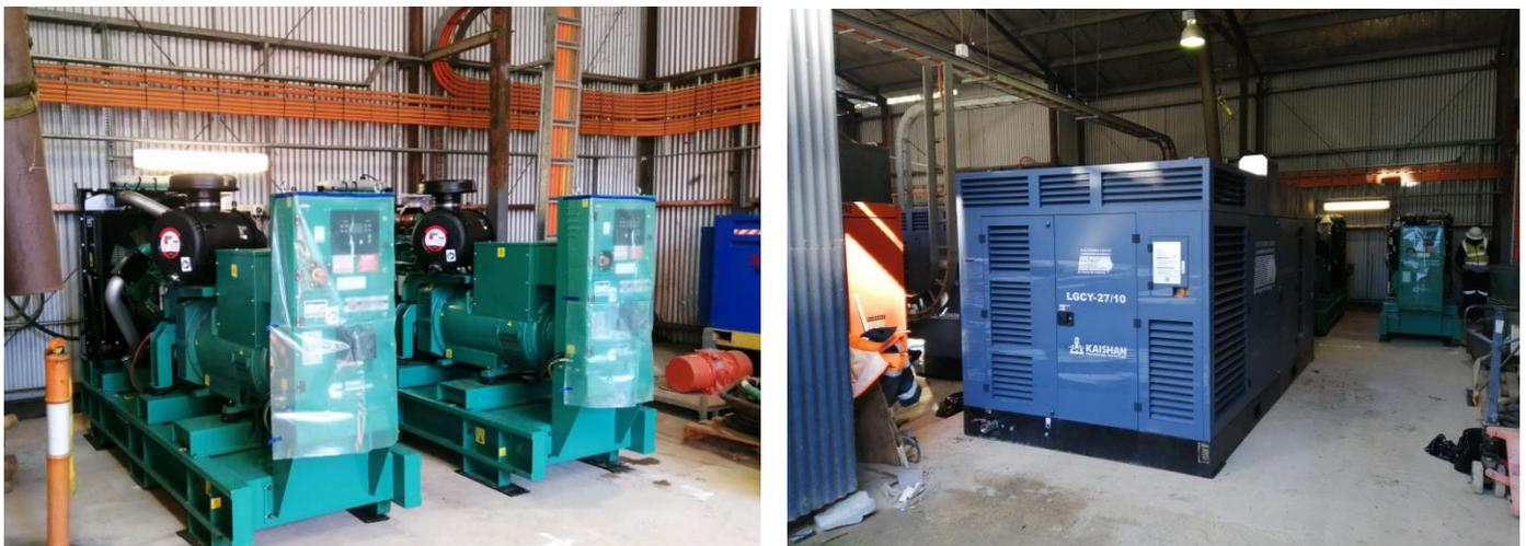
Fig (1): Cummins Generator Units awaiting installation on site (L), Kaishan Air Compressor Units at Morning Star (R)
