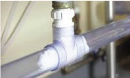
Foaming action extends into drain lines.
