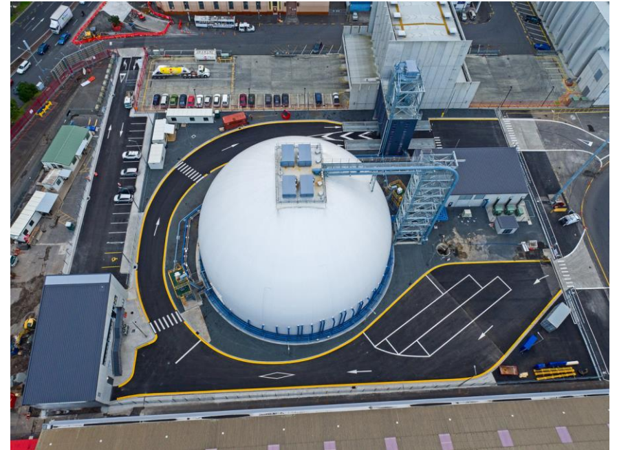
Holcim Bulk Cement Storage Facility (Auckland, New Zealand) with pneumatic loading/Unloading.
