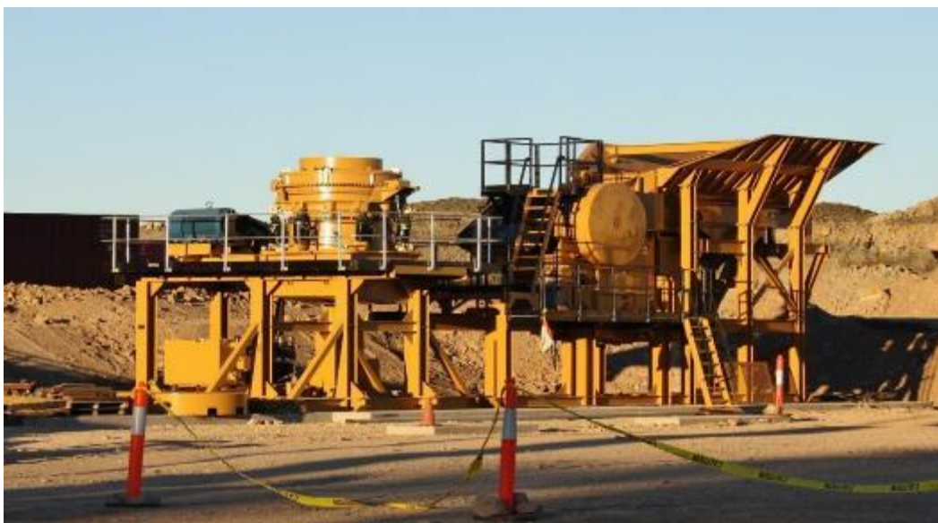
Figure 13: Primary and secondary crushers during installation in 2011.
