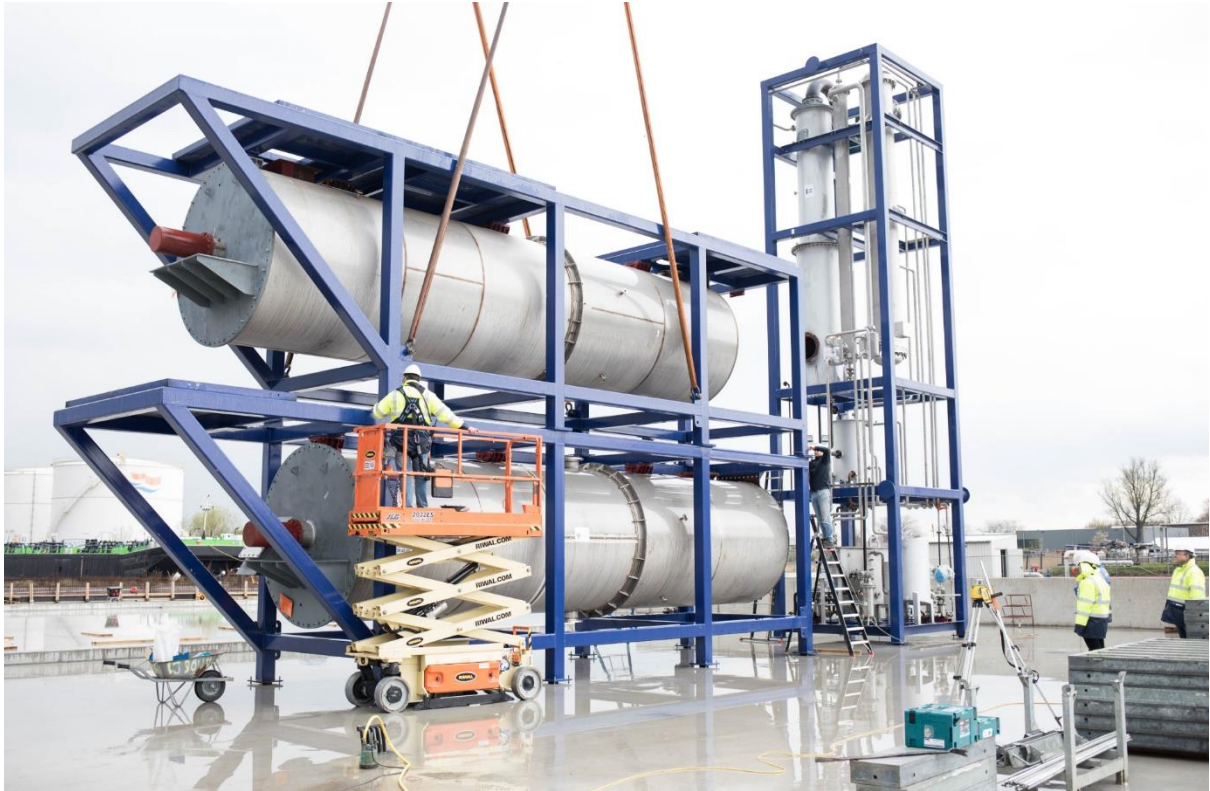
50TPD module successfully transported to the IGES Amsterdam plastic to fuel facility.
