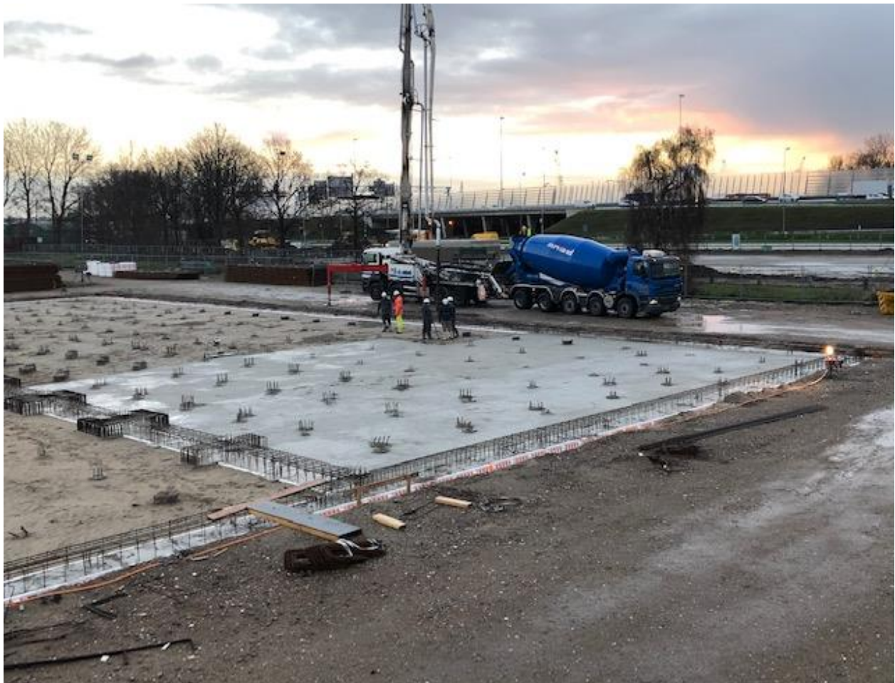
Pouring of the concrete base on site at Amsterdam in December 2018
