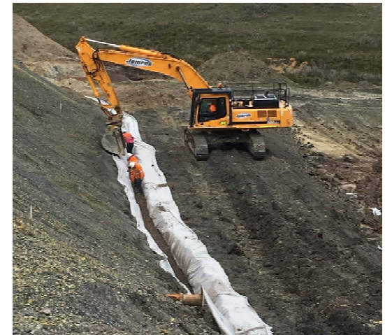
Construction of new Tailings Storage Facility
