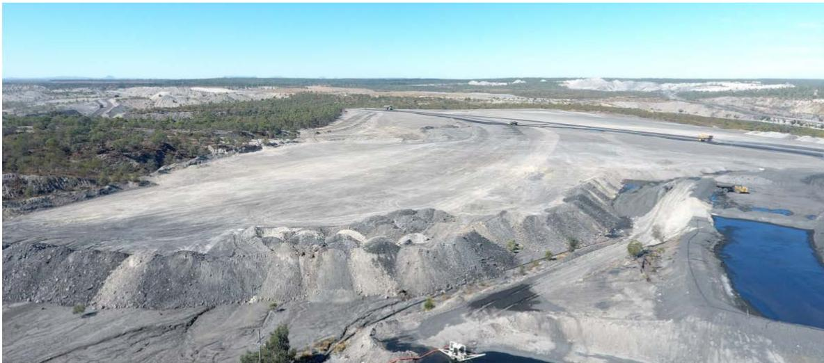
*Image – TSF capping completed, decant calls in bottom right corner.*
