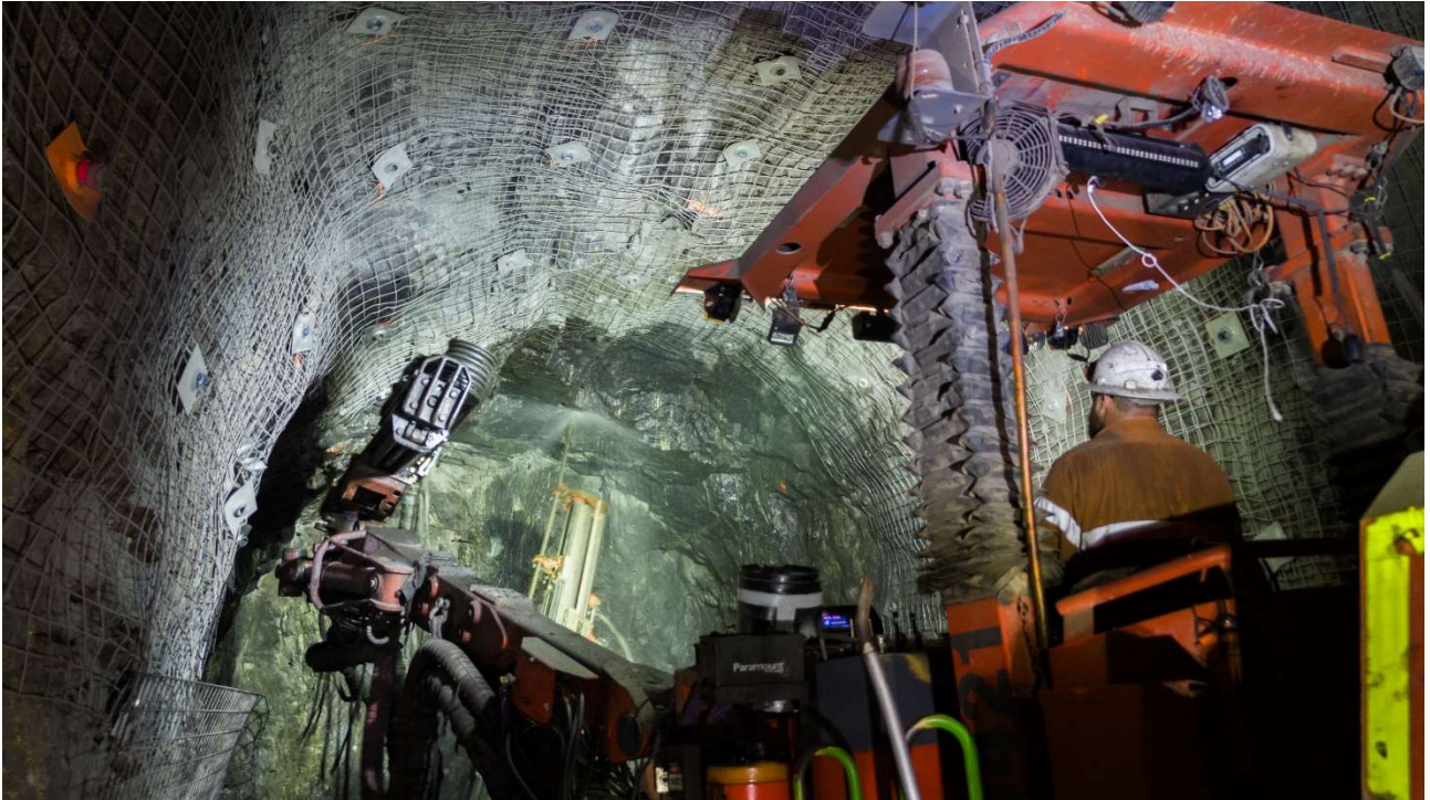
Figure 1 Scaling the backs of an ore drive
