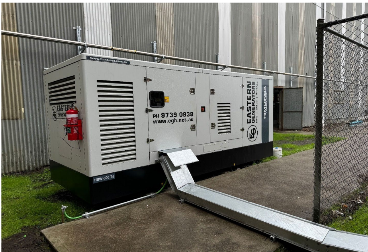
Figure: Emergency Standby Generator installed
