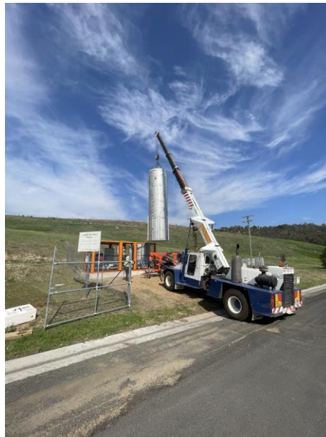
Installation of flare at Bathurst
