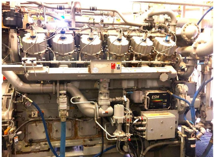
Part of the newly acquired RPGP - Low pressure gas is compressed to sales gas pressure using gas engine driven reciprocating compressors
