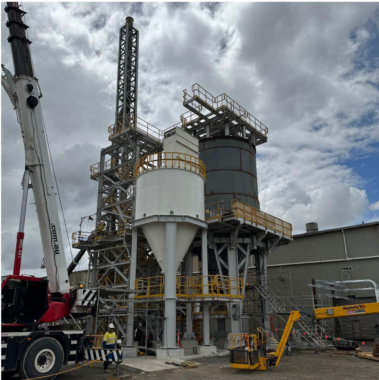
**Figure:** Spray Roaster's reactor vessel & oxide bin installed along with structural steelwork erection complete.
