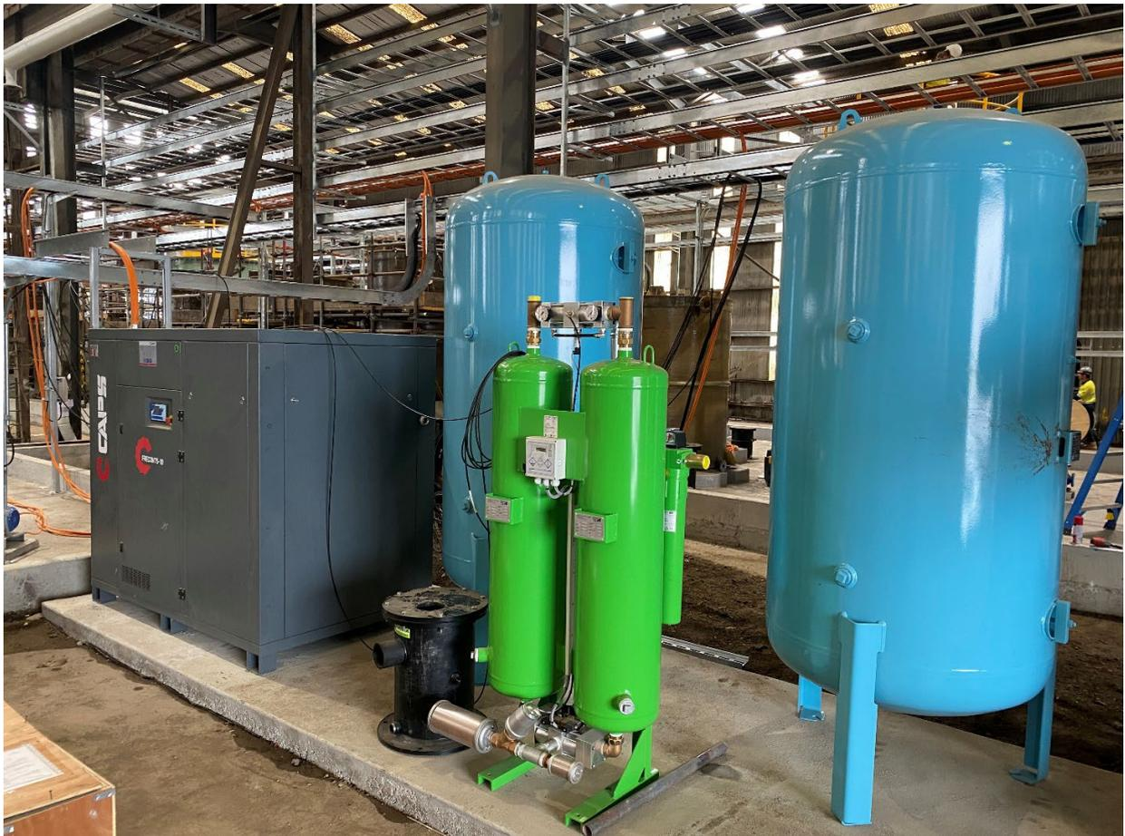
**Figure: Filter area FRP tanks and air compressors installed**
