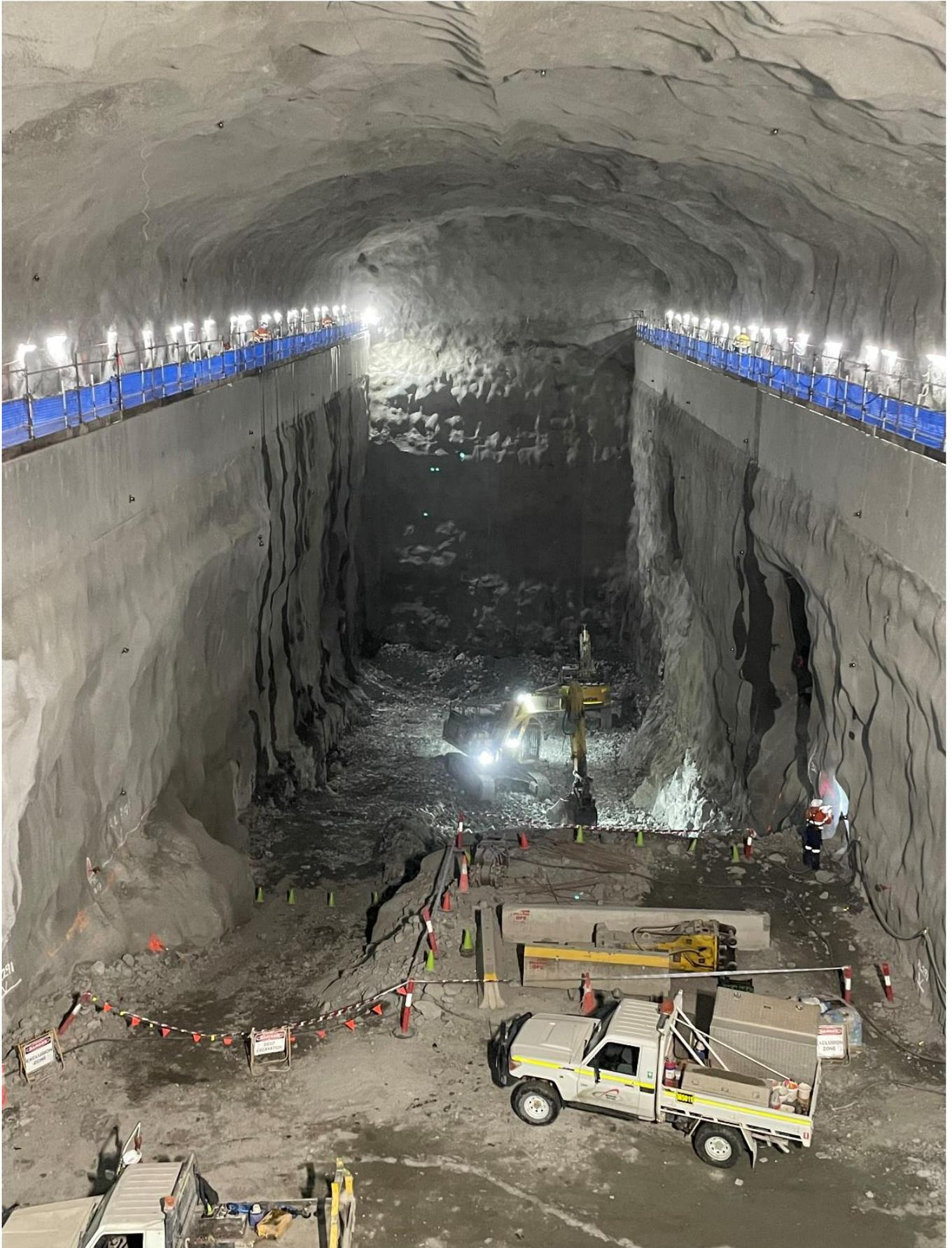
Figure 1: Powerhouse Cavern excavation
