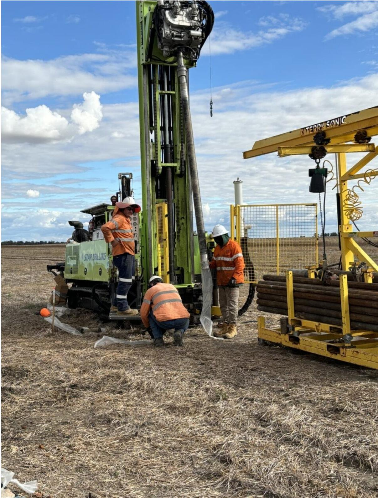
**Figure 2– Geotechnical drilling on proposed Process Plant location, March 2024**
