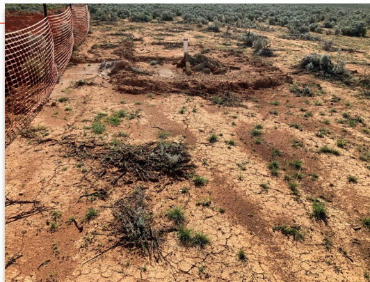
Roll bushes at drill sites, no grading or bulldozing
