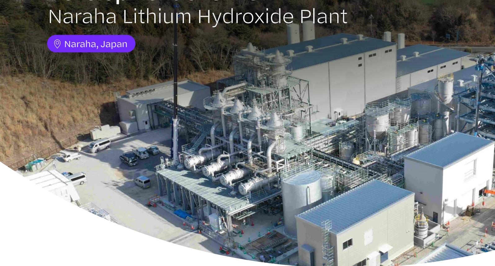
The Naraha Lithium Hydroxide Plant (**Naraha**) is the first of its kind to be built in Japan and is designed to convert technical grade lithium carbonate feedstock into purified battery grade lithium hydroxide. Feedstock for the 10,000 tonne per annum (**tpa**) Naraha Plant will be sourced from the Olaroz Lithium Facility's Stage 2 Expansion that will produce technical grade lithium carbonate.
