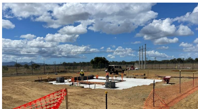
Figure 8: Powerlink works, preparing the bench for the main transformer
