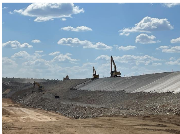
Figure 1: Wises Dam, cement stabilised crusher dust placement Ch4000 - 26 September 2022
