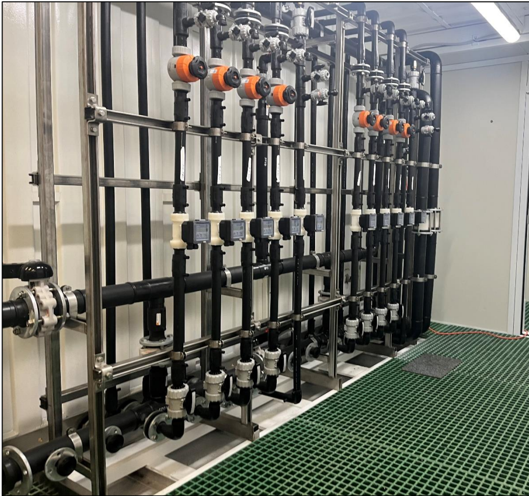
Photo 1: Progress of well house fabrication inside transportable container for Field Recovery Trial pilot plant - off-site fabrication.
