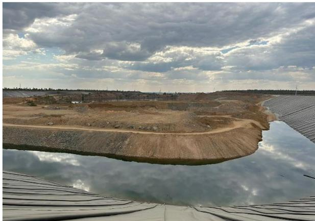
Figure 2: Wises Dam liner installation
