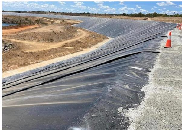
Figure 3: Wise Dam liner installation
