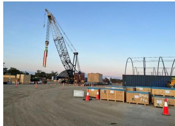
Figure 5: Unloading of one of the main inlet valves at the laydown area on site
