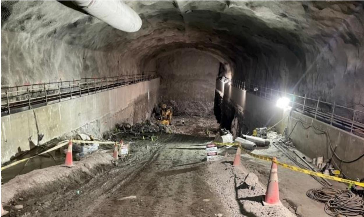
Figure 1: Powerhouse Cavern excavation
