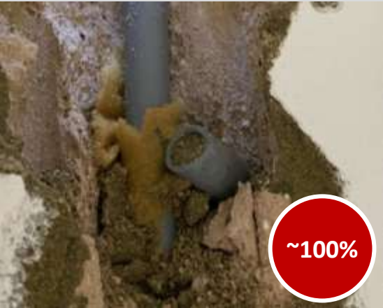
Lagging not impermeable (and at times non-existent)
