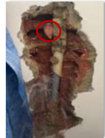
Inadequate movement and damage to pipe caused by pegging left in chase
