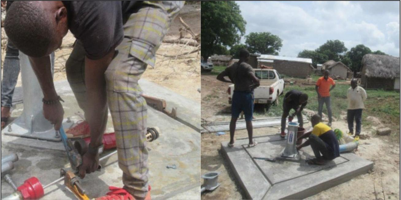
**Figure 15: Installation of water well pump mechanism**
