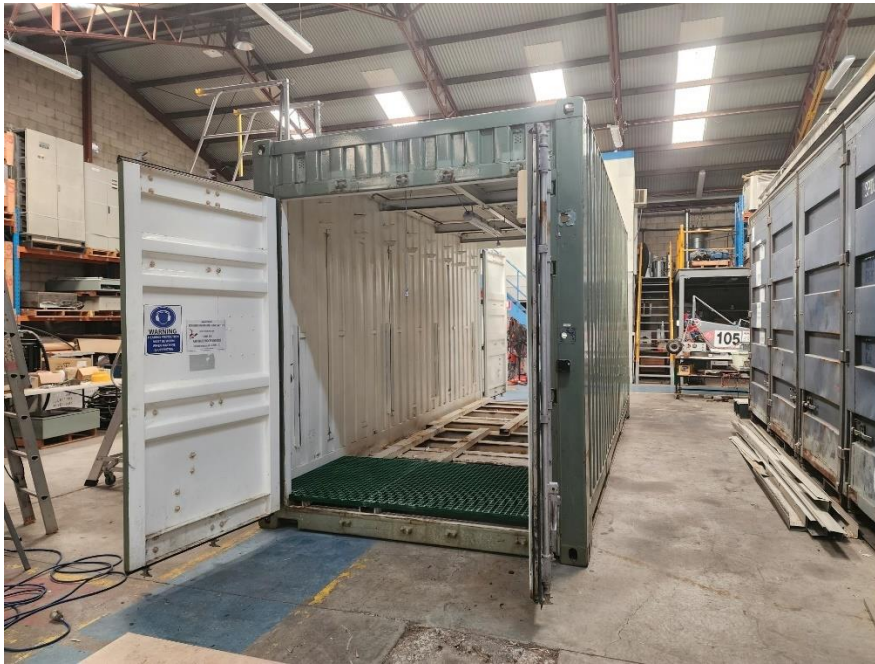
Figure 2: Floor bunding being installed in the FRT wellhouse container.
