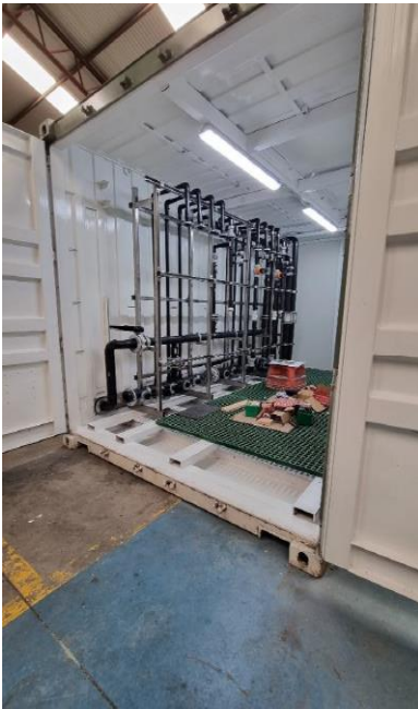
Photo 1 and 2: Progress of well house fabrication inside transportable container for Field Recovery Trial pilot plant - off-site fabrication.
