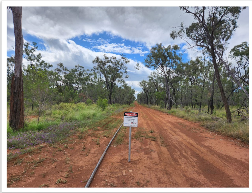
Temporary overland pipeline connecting Rednook-1 to gathering – Dec 22
