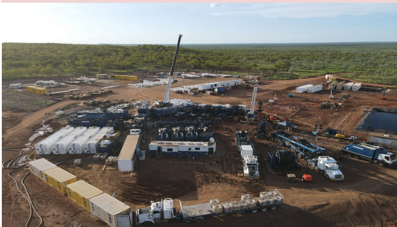
Schlumberger hydraulic stimulation operations on C-3H well
