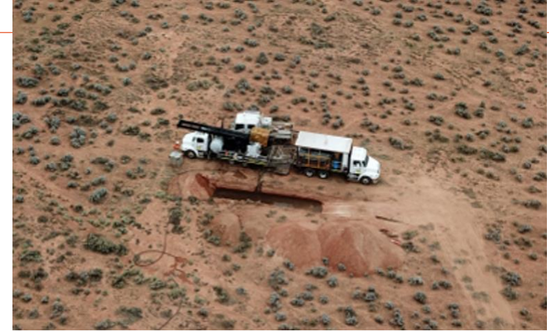
Topsoil separation, access track rolled not graded
