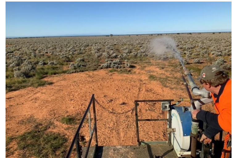
Hydroseeding holds soil and seed in place
