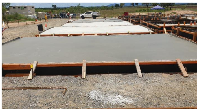
Figure 7: Megapack foundations
