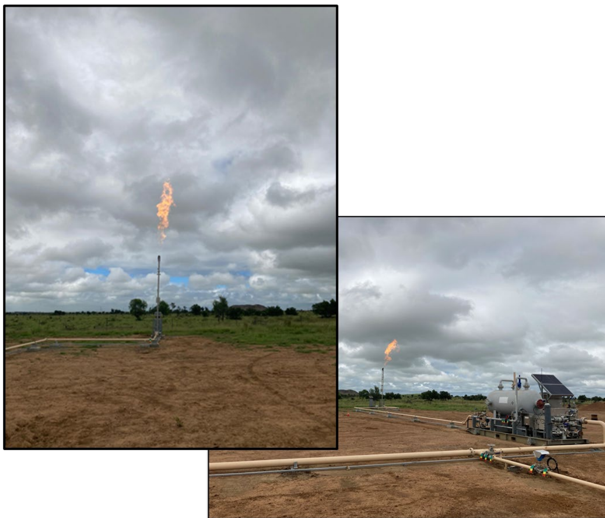
Figure 1: Sapphire 6 flare stack with blow down gas flaring during surface facility commissioning
