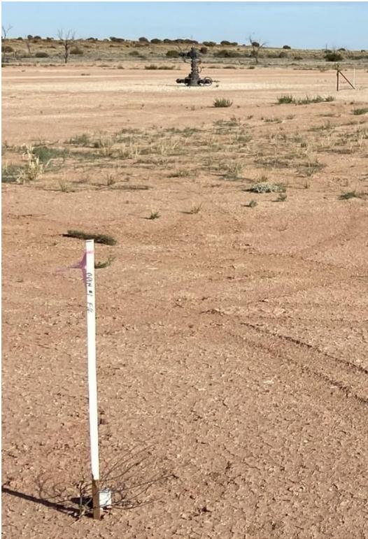
**Odin flowline right-of-way marker with Odin-1 wellhead in the background**
