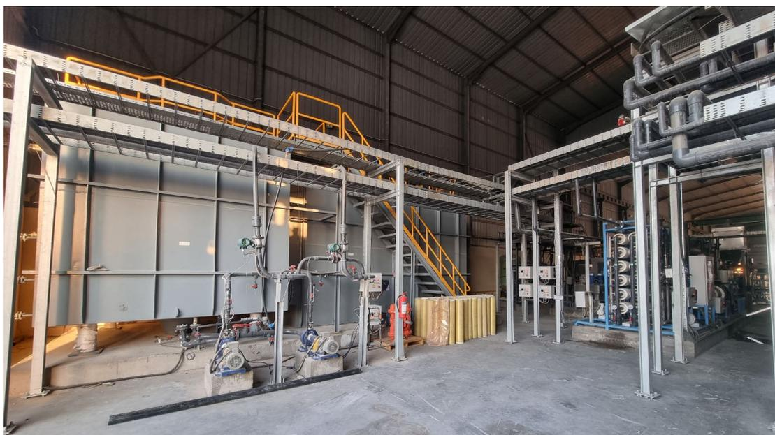
*Photo of the brine recovery circuit of the HIROX<sup>®</sup> plant*
