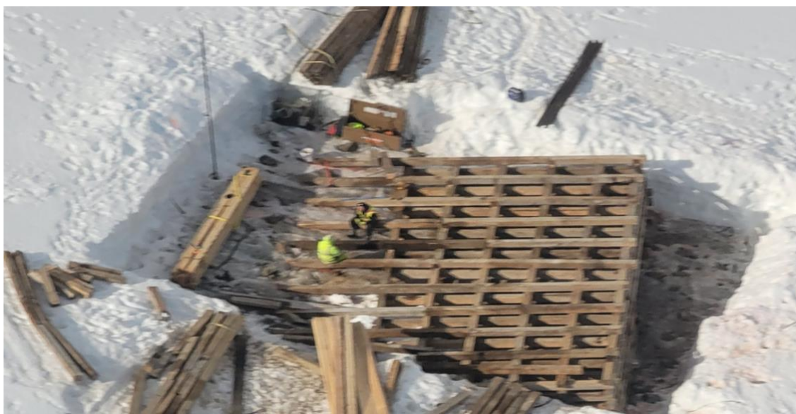
Figure 4. New pad constructed in the valley for drilling the 600m link zone as per Figure 6 below
