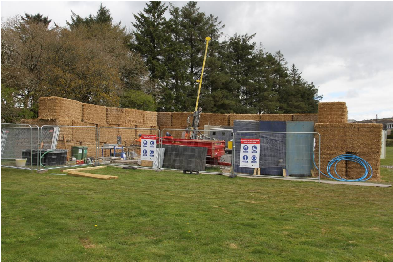
Figure 6 - Drilling underway, with bales successfully used for acoustic mitigation
