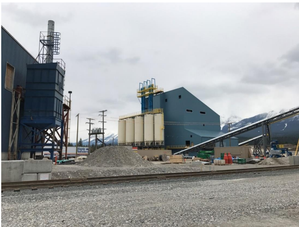
External silos and bucket elevators installed
