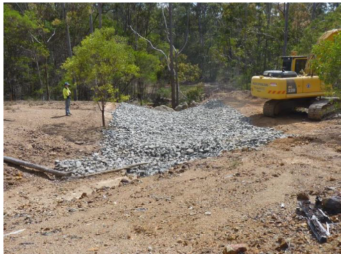
Plate 2: Ongoing erosion control works completed.
