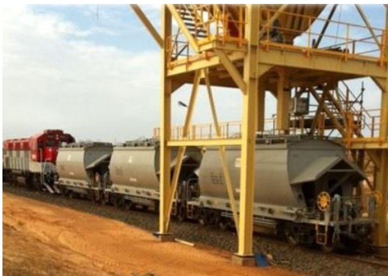
Figure 7.1 Train loader overhead hopper
