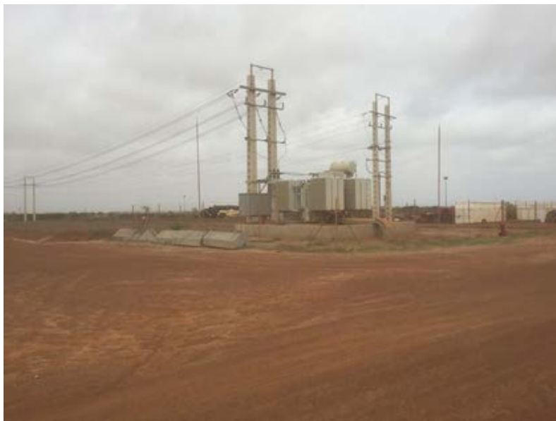
Figure 6.5 33 kV Transformer and overhead line
