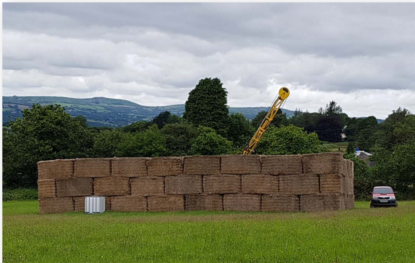
Straw bale noise screen to minimise disturbance
