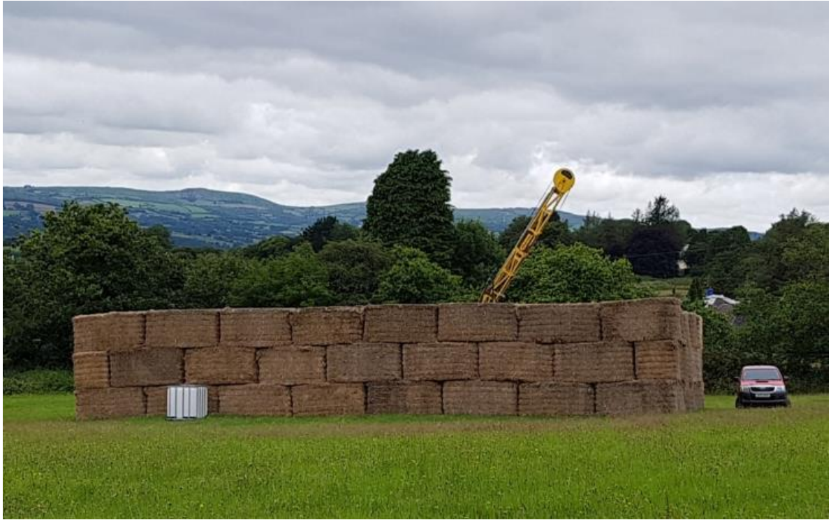
Figure 7 - Straw bale noise-screens minimise disturbance from drilling
