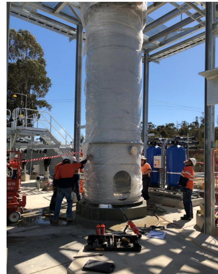
Ion-exchange columns installed at Fosterville Gold Mine
