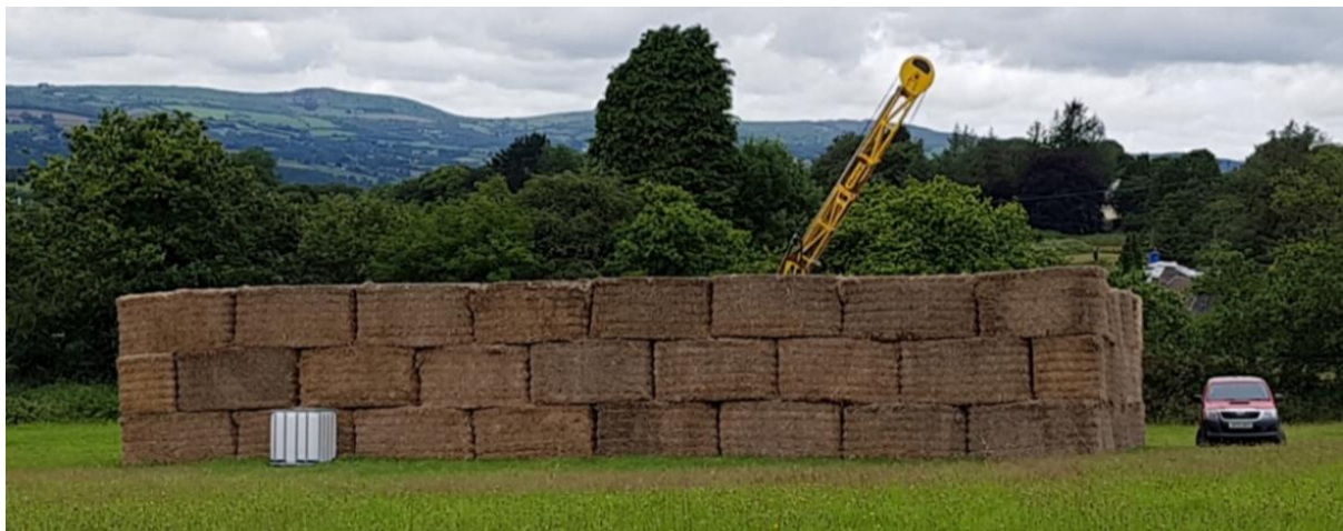
Figure 6 - Drilling underway, with bales successfully used for acoustic mitigation
